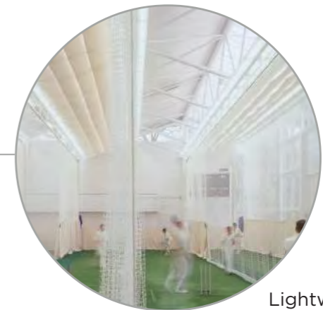
Simple gable steel framed roof
